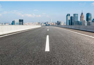
Wide access road with durable surface
